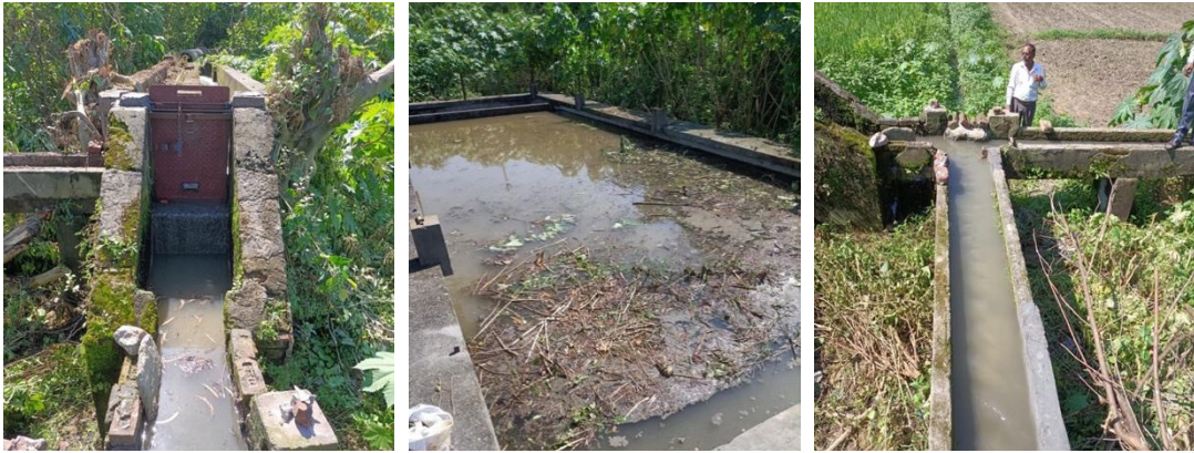
Sewage at the inlet
