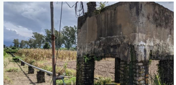
Tube well installed at the Sewage farm by private party to maintain clean water supply for crops
