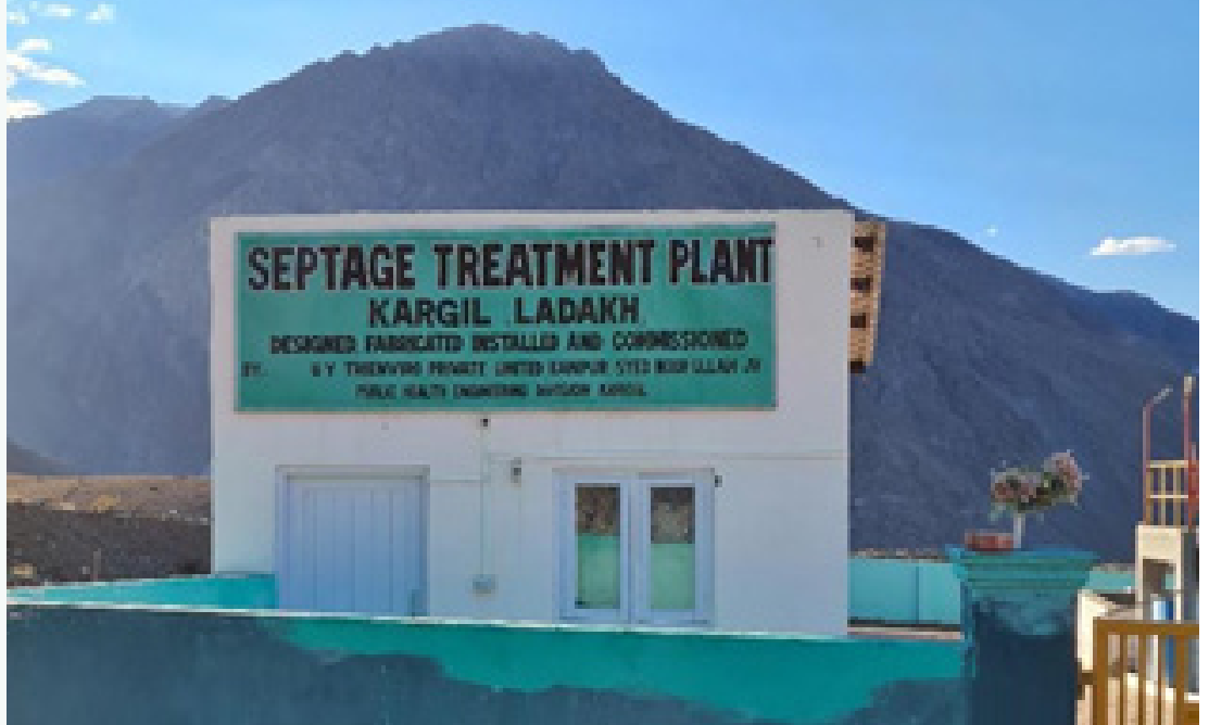
Figure 15: Septage Treatment Plant, Kargil
