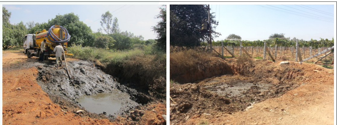
Faecal sludge is emptied into a storage pit. This is covered in a layer of soil and cow dung/sheep dung, and allowed to dry and compost for 3-6 months, before application on land.
