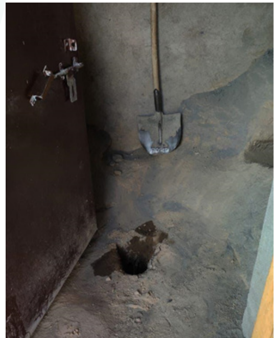
Figure 16: Typical dry toilet, Kargil
